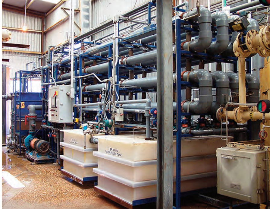
A Duraflow Tubular Membrane system installed and running.
